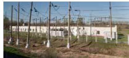
Improving the efficiency of energy recovery
